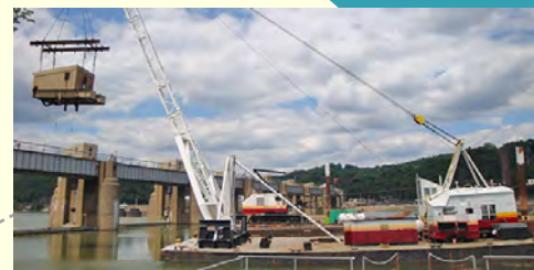
Emsworth Locks and Dam
