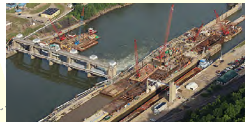
Charleoi Locks and Dam
